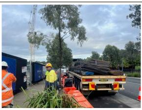
Photos 8-12: Pedestrian diversions were in place and safety barriers had been placed around footpaths. Traffic controllers were in place to guide pedestrians around the site. Approved work zones on Conferta Ave and Andalusian Drive were in use pedestrian diversions in place.
